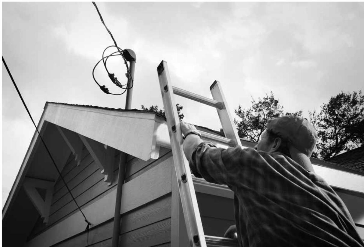
pressure from below — as from a hose or sprayer. And, if you slip and fall against the service mast, pulling wires loose, you risk being severely shocked or electrocuted by exposed wires.
