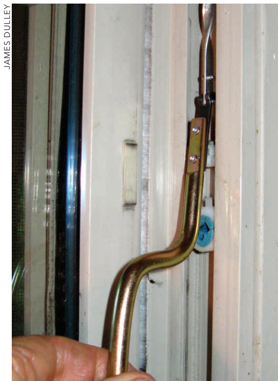
DO-IT-YOURSELF: Other than a screwdriver, the spring-tension charging tool, designed just for the tilt-type spring end, is all you'll need to fix a window that just won't stay open.
